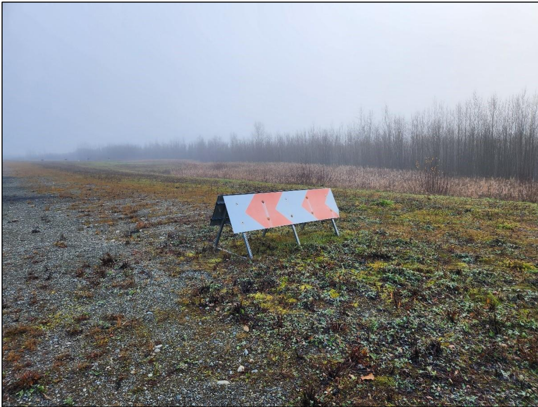
Figure 8: Runway 04/22 RSA Non-frangible Threshold Markers
